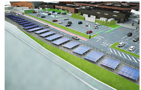
Installed solar panels (Fukaya-Hanazono Premium Outlets)
