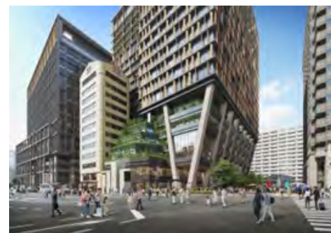
CLT panels and extensive green spaces on the lower floors of the building
