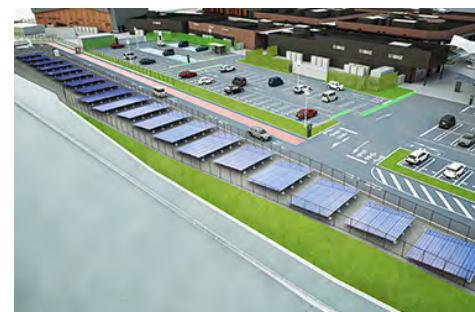
Installed solar panels (Fukaya-Hanazono Premium Outlets)
