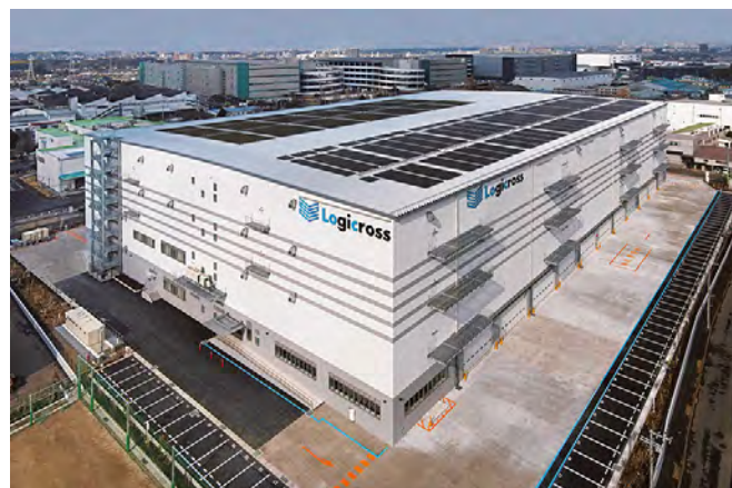
Logicross Zama Komatsubara (completed in March 2022)
