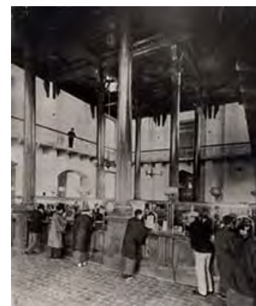
Former bank lobby
