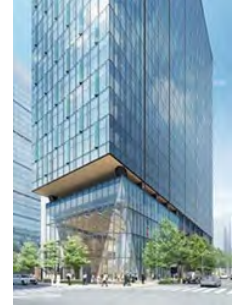
Otemachi Gate Building
