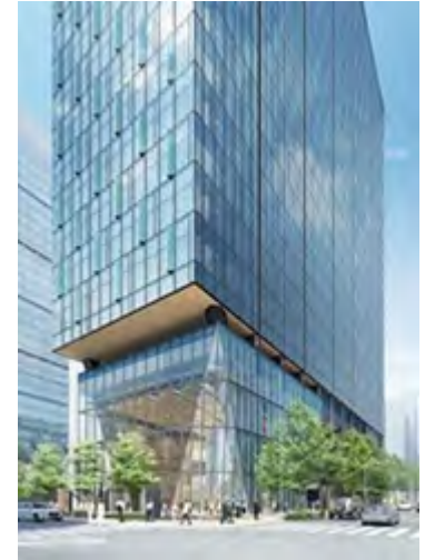
Otemachi Gate Building
