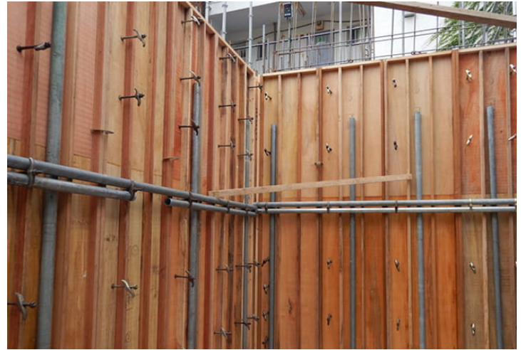
Example of formwork panels in use
