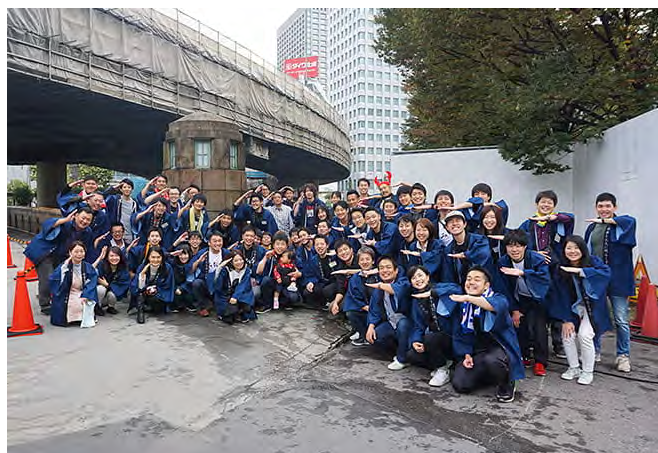
Tokiwabashi bridge clean-up, the first event in the Japan Nationwide Bridge Project
