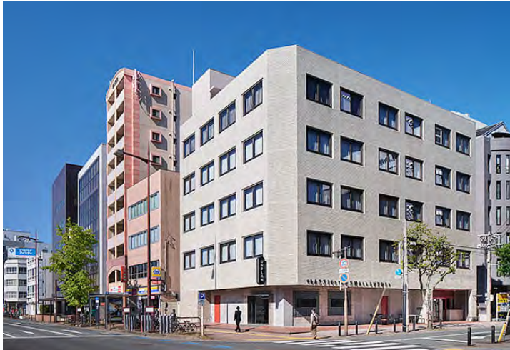
Building exterior after renovation
