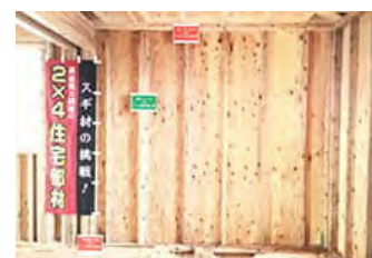
Example of construction of wall frames using Japan-grown timber
