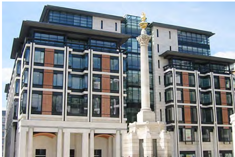
Photo from the building front
