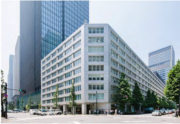
Otemachi Building before renovation
