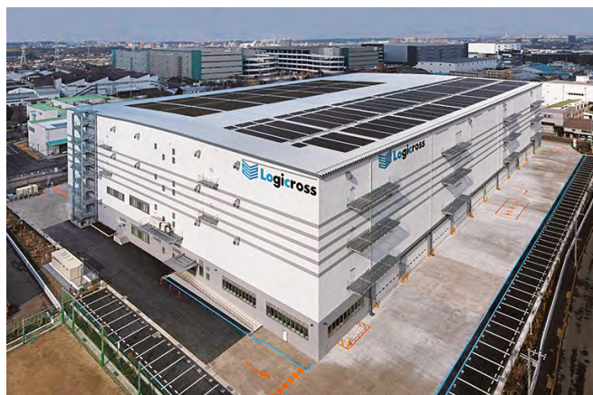
Logicross Zama Komatsubara, Completed March 2022
