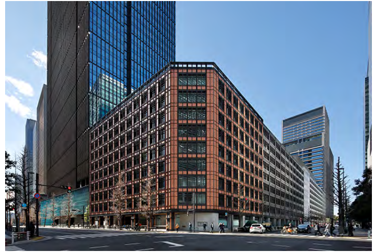
Otemachi Building after renovation
