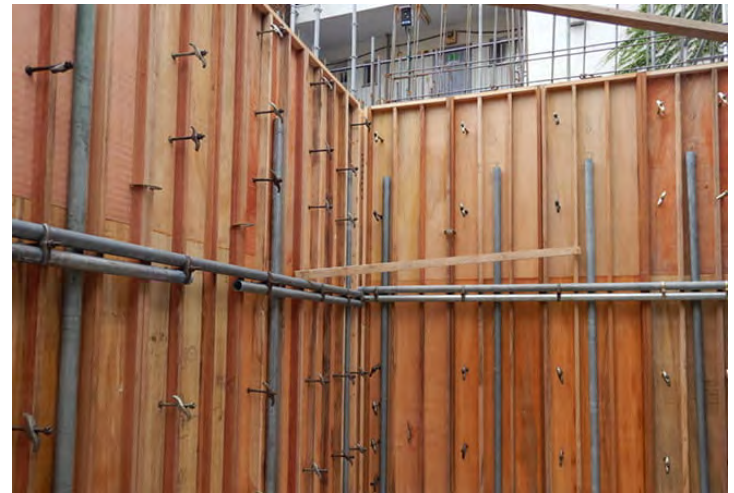
Example of formwork panels in use
