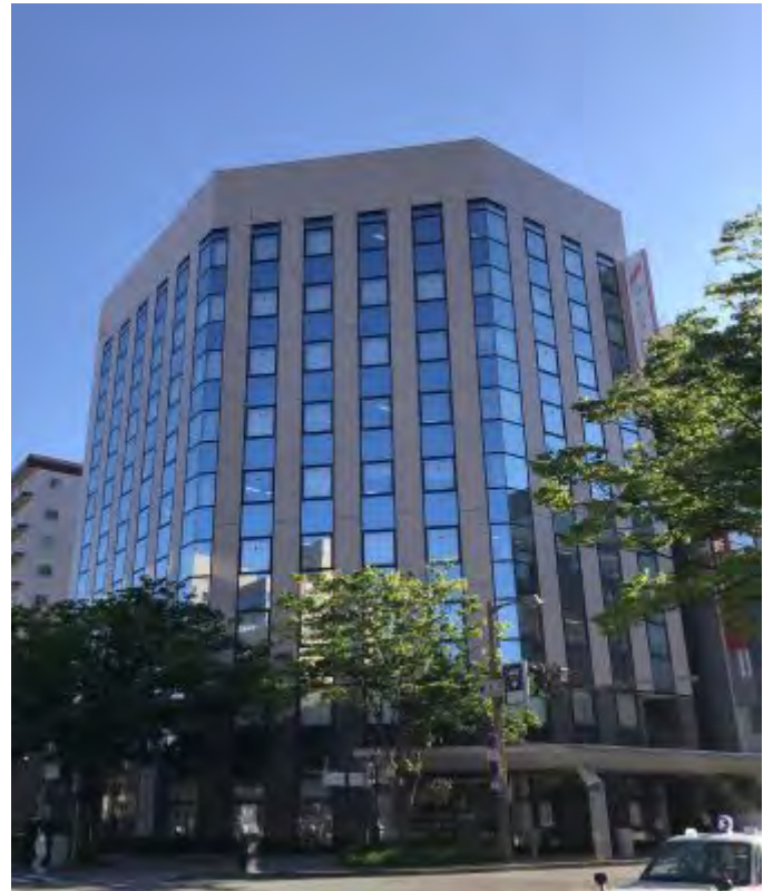
Daido Seimei Niigata Building
