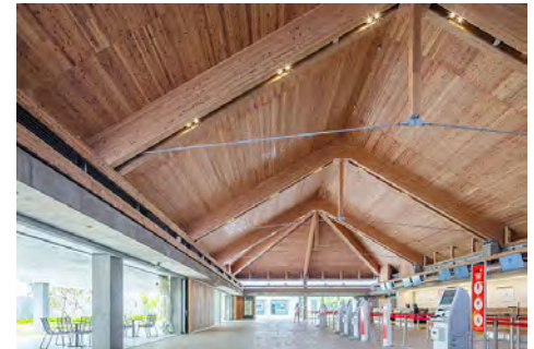
Check-in lobby using CLT as structural material for the roof
