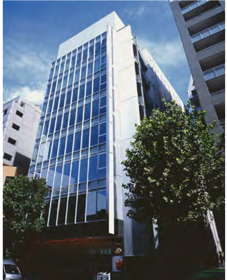
JRE Higashi-Gotanda 1-Chome Building
