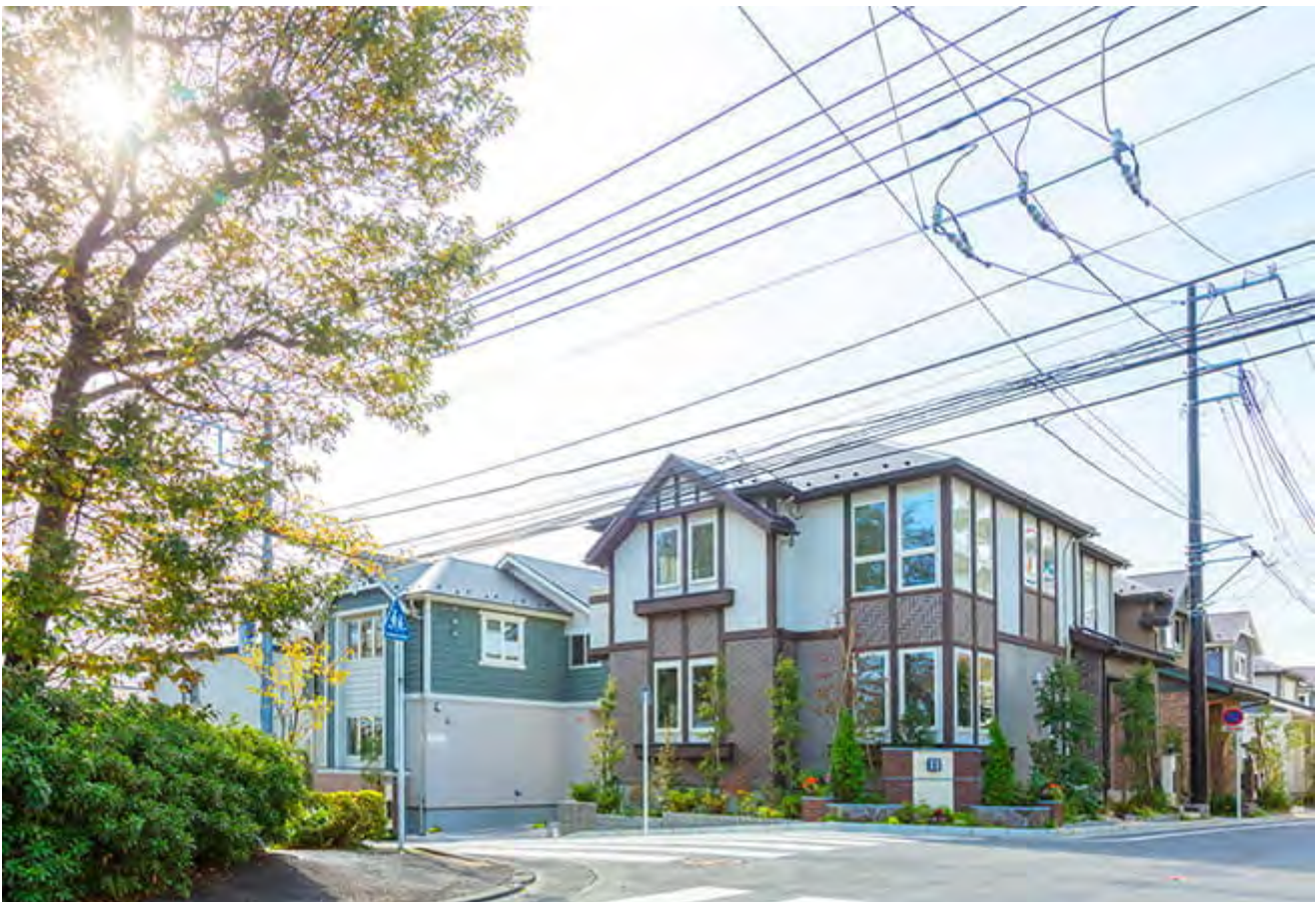
Exterior of The Parkhouse Stage Higashitotsuka, where ENE-FARM was first introduced
