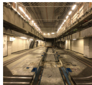
Former rotary press room (before renovation)
