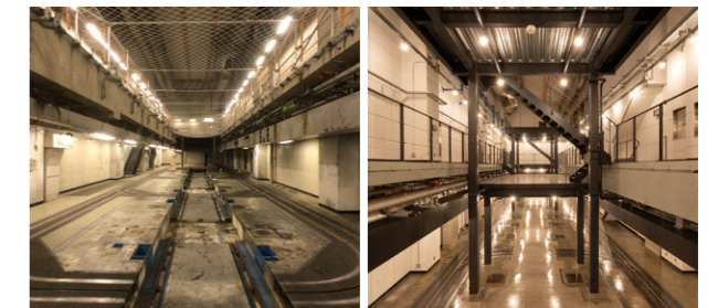
Former rotary press room (before renovation)
