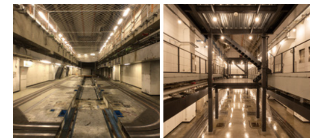
Former rotary press room (before renovation)
