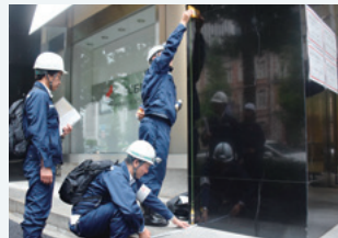
Emergency safety checks of buildings
