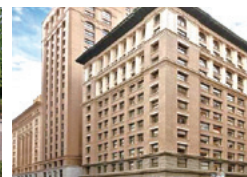
115 Sansome, San Francisco, California (offices)
