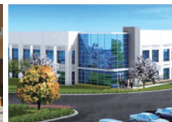
I-210 Logistics Center II, Rialto, California (distribution facility)
