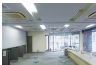
Before renovations (first floor)
