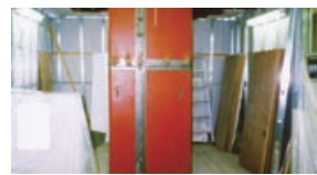
Beam and column reinforcement
