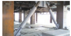
Examples of seismic damping devices (left: brace type; right: wall type)
