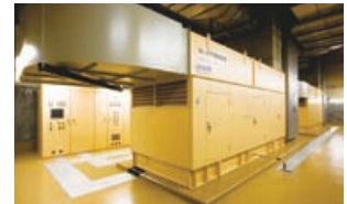
Emergency power generators
