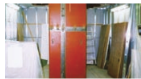
Beam and column reinforcement
