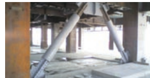
Examples of seismic damping devices (left: brace type; right: wall type)
