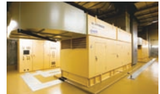
Emergency power generators
