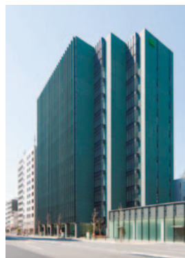
Midori Anzen Co., Ltd., headquarters building (Shibuya Ward, Tokyo)
