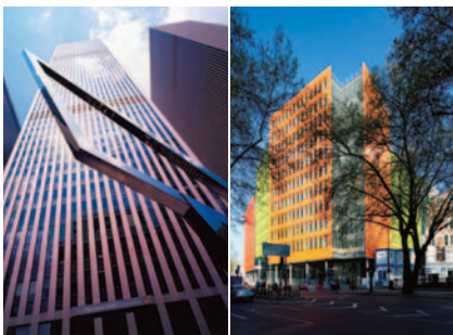
The McGraw-Hill Building Central St Giles
