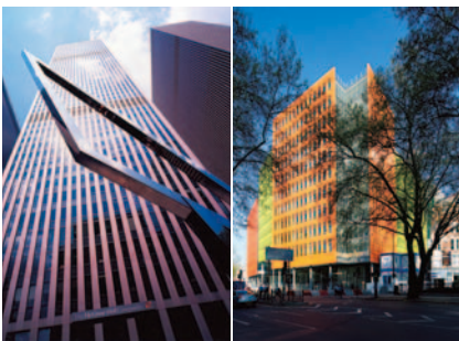
The McGraw-Hill Building Central St Giles
