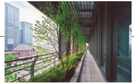
Rooftop greenery Air temperature goes down as plant and soil moisture evaporates, and the greenery also helps shield the building from heat.
