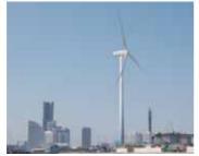
Power-generating windmill operated by the Yokohama Wind Energy Project (rated power output of 1,980 kW)
