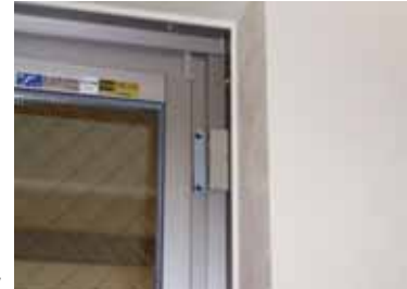
Magnetic sensor on a window
