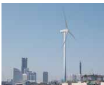
Power-generating windmill operated by the Yokohama Wind Energy Project (rated power output of 1,980 kW)
